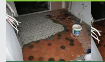
I then dragged a wet towel over it to pick up as much of the excess grout as possible. I then cleaned the tiles using a bucket of water, a sponge and a green scrubbing pad.
