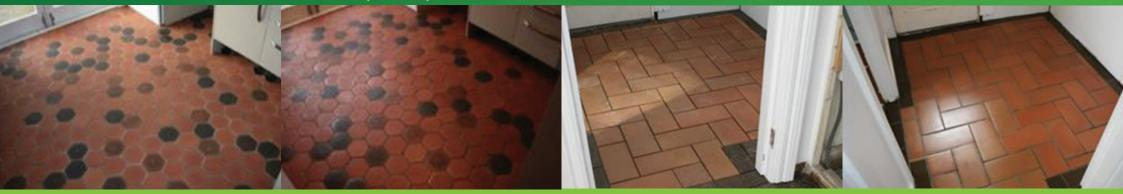
Notice how the grey marks have gone off the tile. Also note that the grout joints have become discoloured. When you put the second coat on pay attention to the joints and you will find they go an even colour at this stage. The finished look should be like my laundry which is shown above
