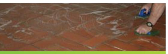
Once the tiles are wet with clean water, you can then wash them with the acid/water mix. You need a big commercial green pad to do this as shown in the photo above.
