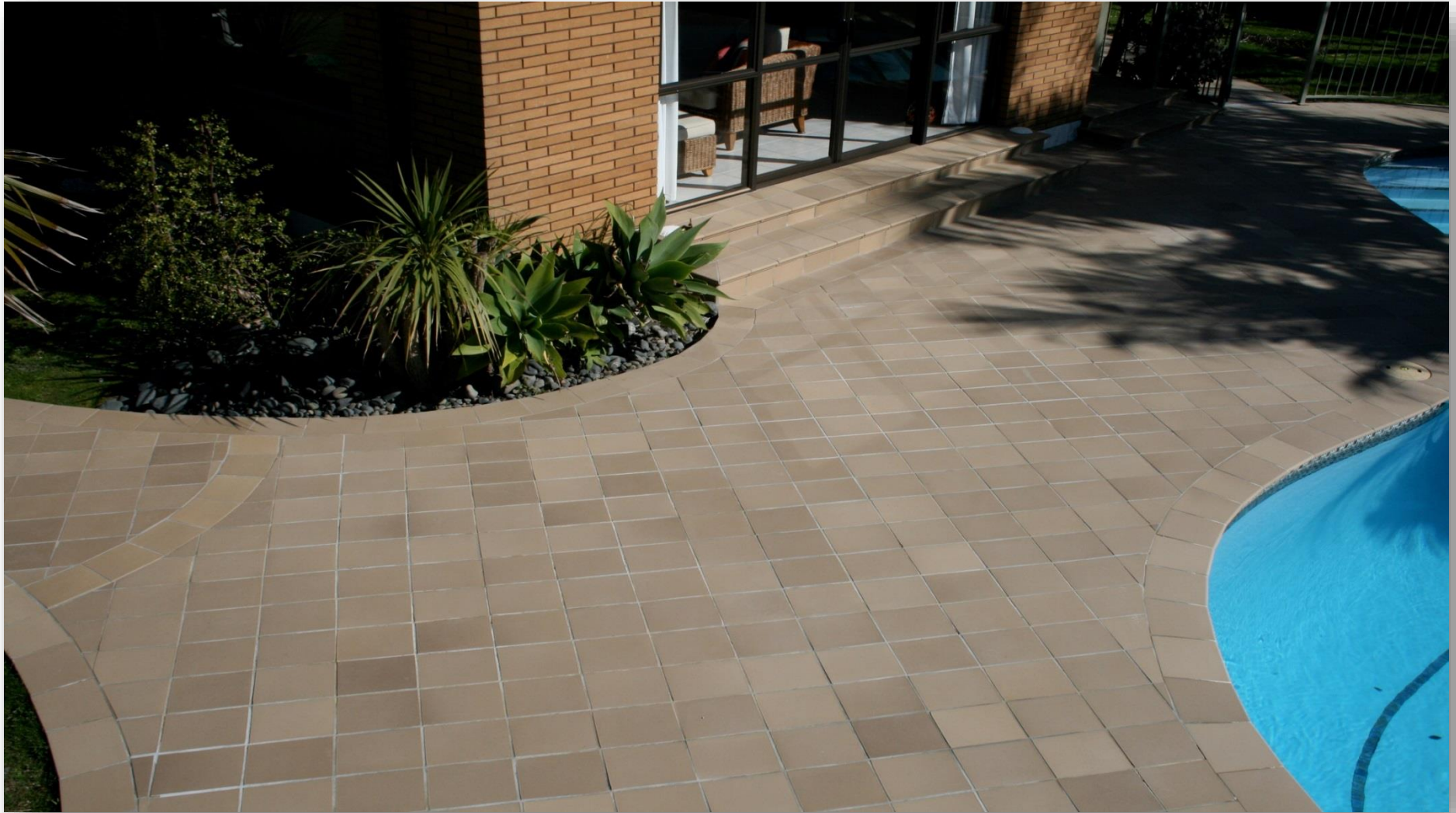
"Run of Kiln" Doeskin coloured terracotta tiles
