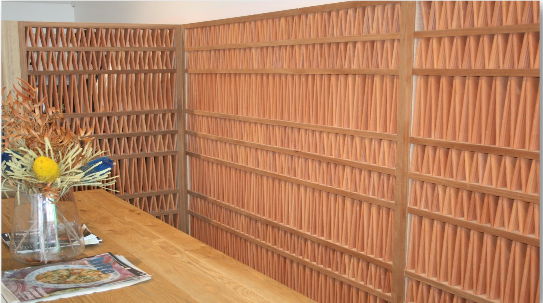
Terracotta tiles used as a Café feature wall
